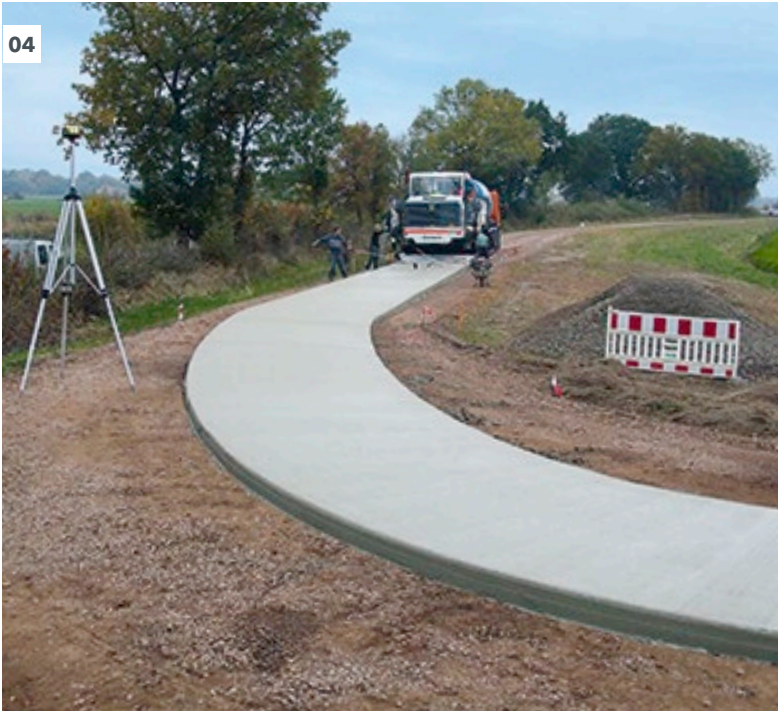
03 - 04 The high-quality machine control system guarantees perfect straight-ahead travel and precise steering in bends.
