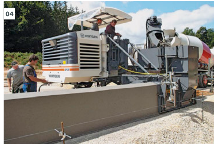
04 - 05 The mold can be mounted on the left or right – modification is completed within an extremely short time.
