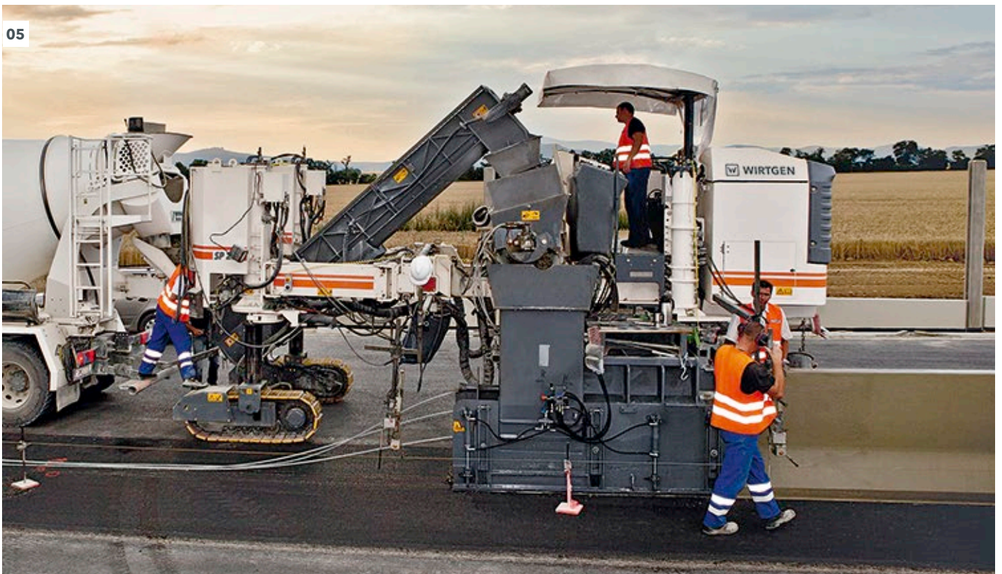
04 - 05 The mold can be mounted on the left or right – modification is completed within an extremely short time.
